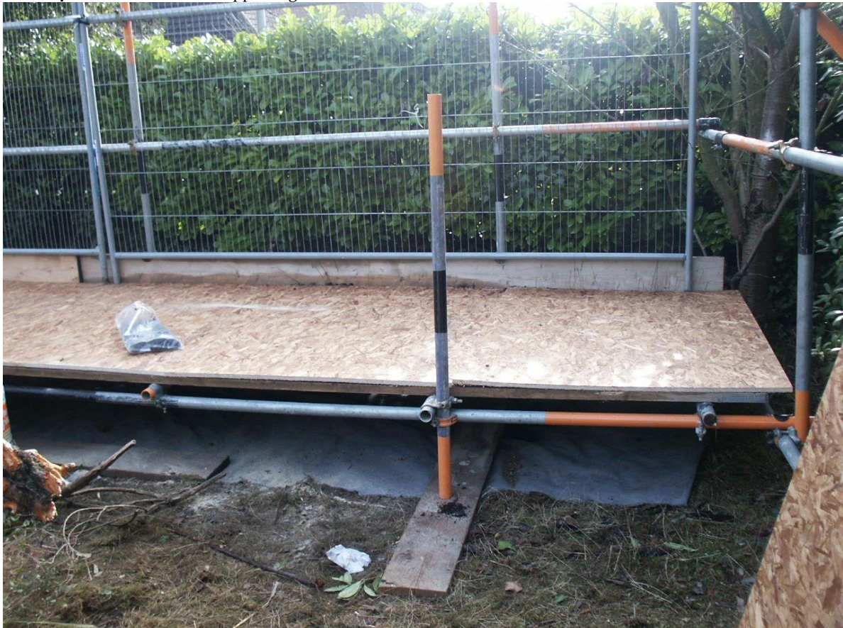
Photo 4 Scaffold framework supporting wooden boards
