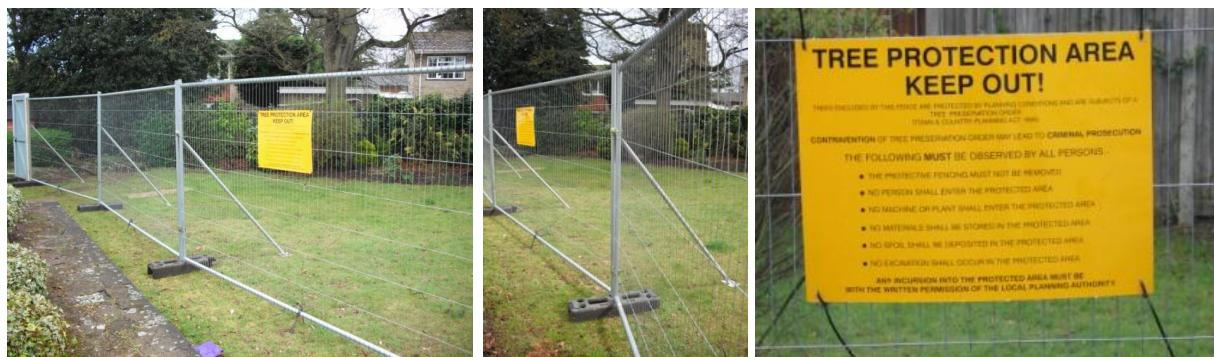
It may *in some cases* be acceptable (e.g. on smaller sites) for rubber or concrete 'feet' at the base of heras fencing to be pinned to the ground or for short outriggers to be attached to the fencing and pinned to the ground in lieu of a full scaffold framework.
