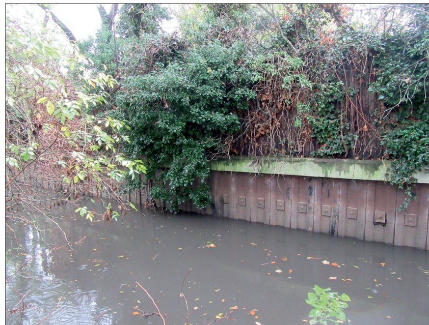
Photograph 4: Showing the concrete retaining wall alongside the Yeading Brook.
