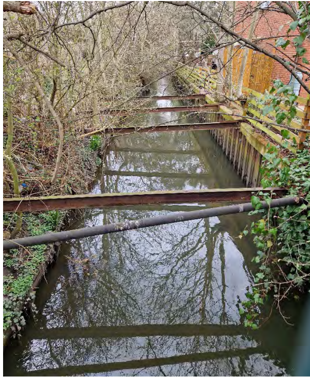
Plate 7: Photograph of Yeading Brook to the west of the site. The sheet piled wall to the side of the brook can be clearly seen.
