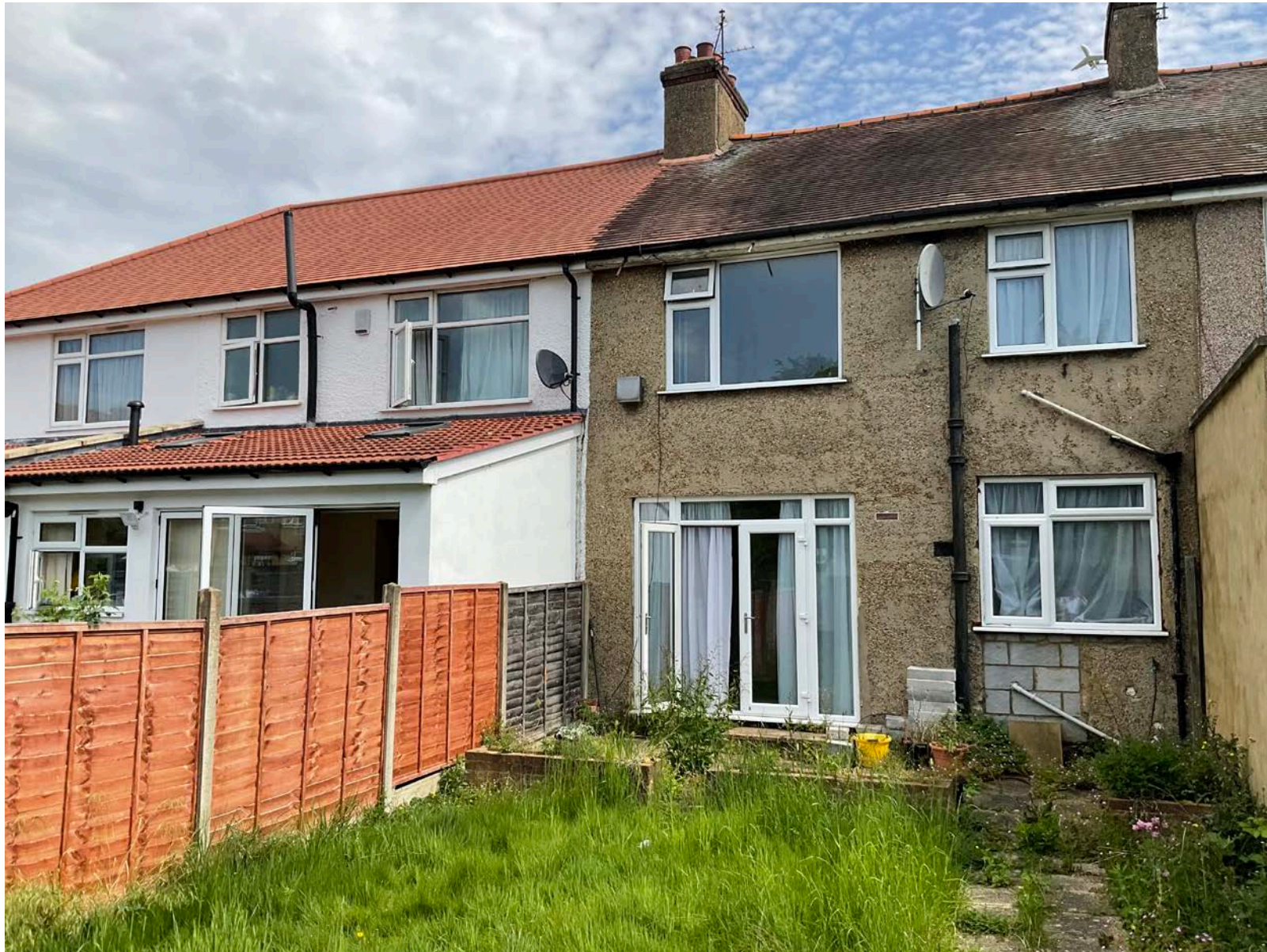
SITE PHOTOS: 80, Ryefield Avenue, Uxbridge, UB10 9BZ
