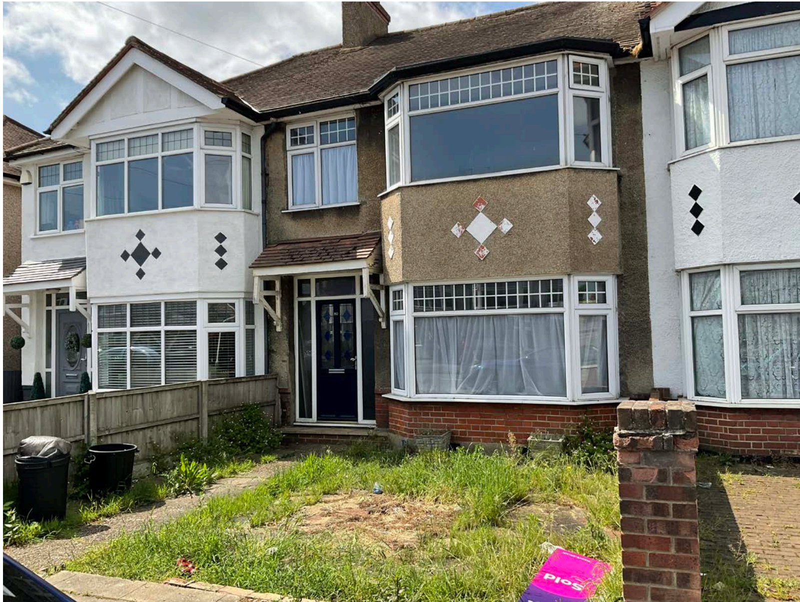
SITE PHOTOS: 80, Ryefield Avenue, Uxbridge, UB10 9BZ
