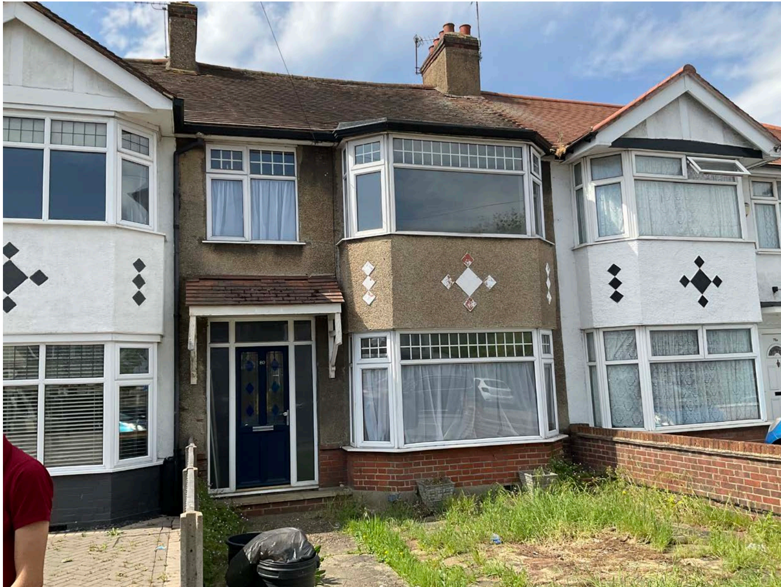
SITE PHOTOS: 80, Ryefield Avenue, Uxbridge, UB10 9BZ
