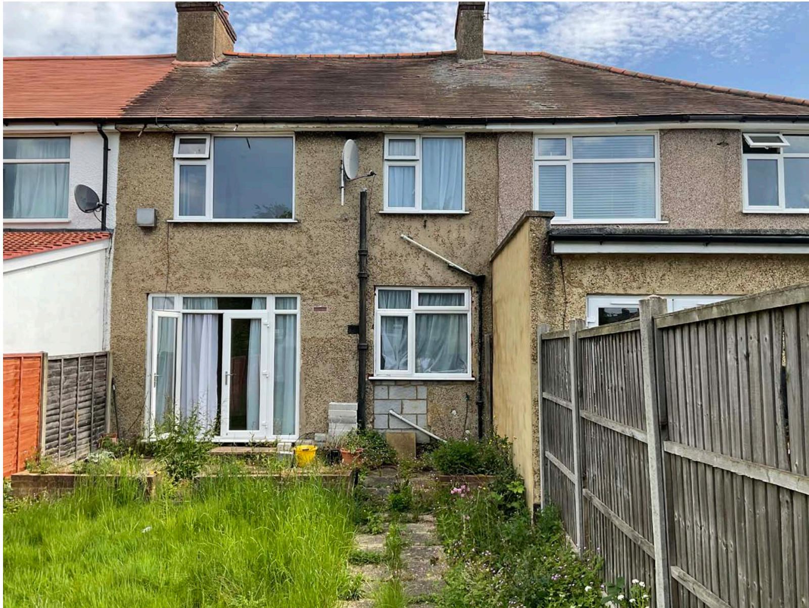
SITE PHOTOS: 80, Ryefield Avenue, Uxbridge, UB10 9BZ
