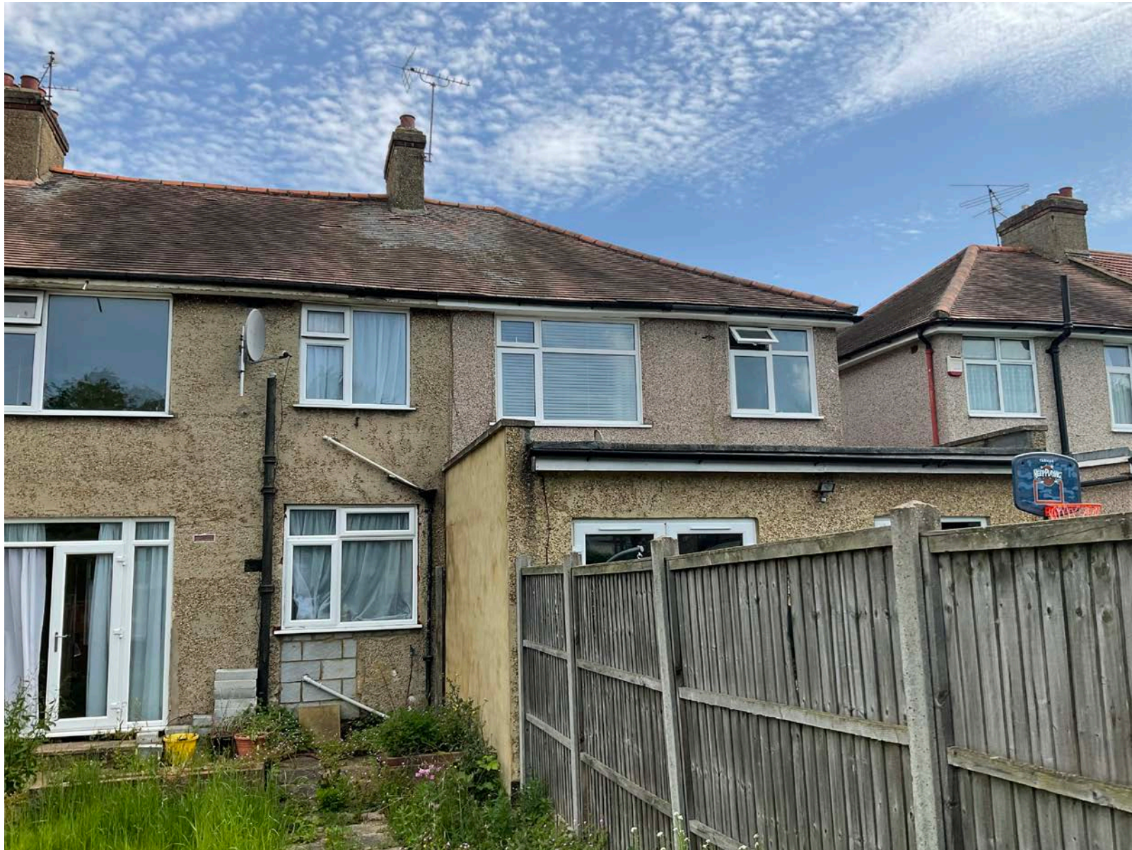
SITE PHOTOS: 80, Ryefield Avenue, Uxbridge, UB10 9BZ
