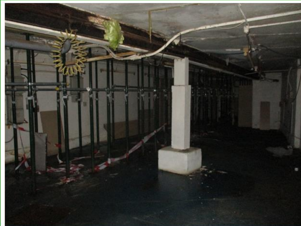
Photo No.6: Facing east from the western side of the rear room showing structural pillaring and acrows
