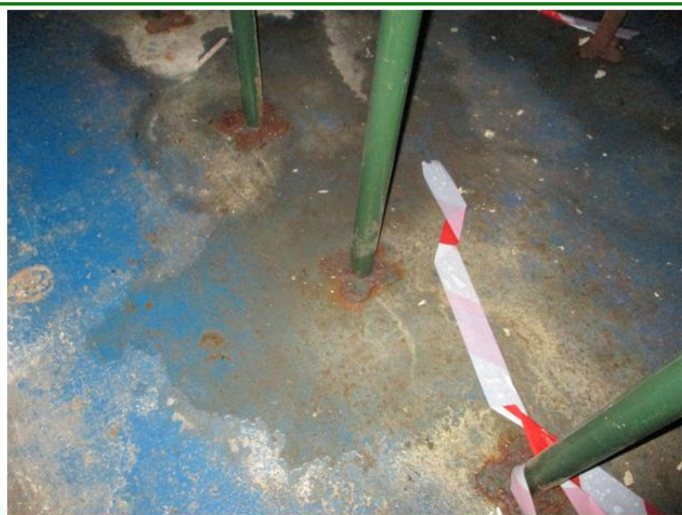
Photo No.9: Shot showing pooling water on concrete flooring
