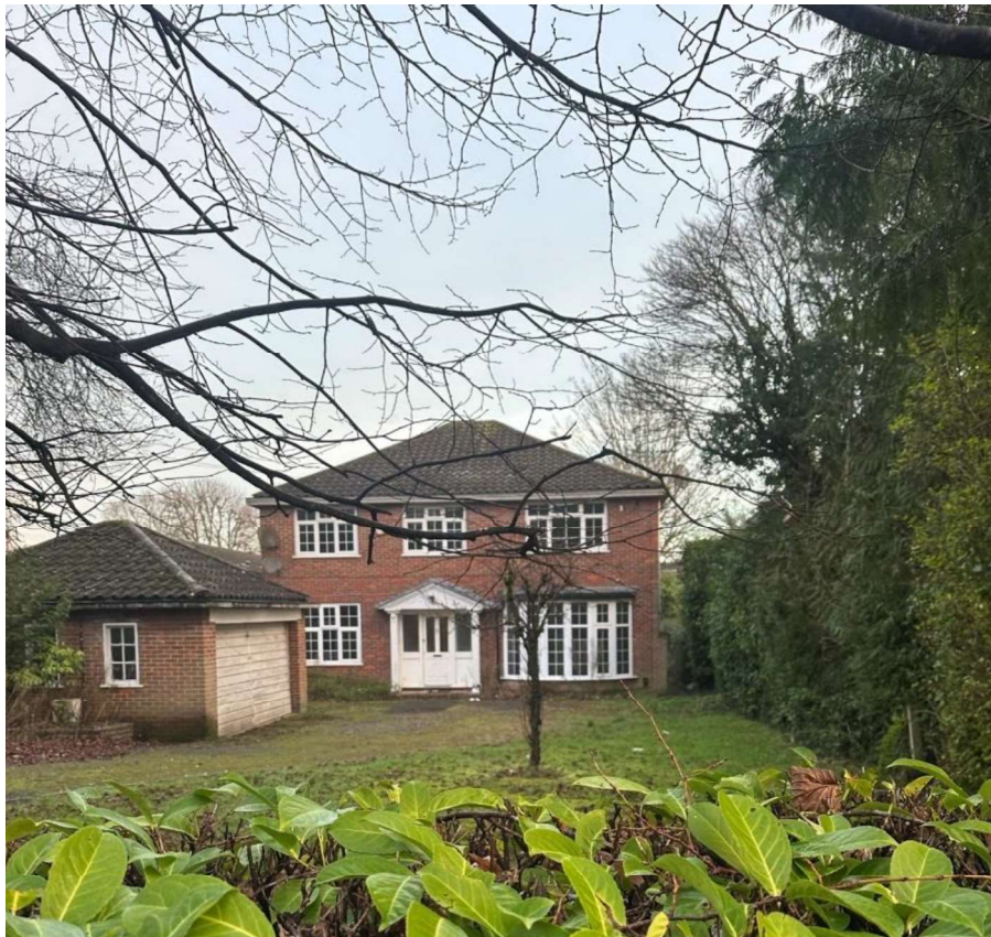
Figure 3: Application Property and garage
