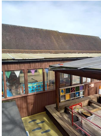
Photo 2 lean to roof junction
