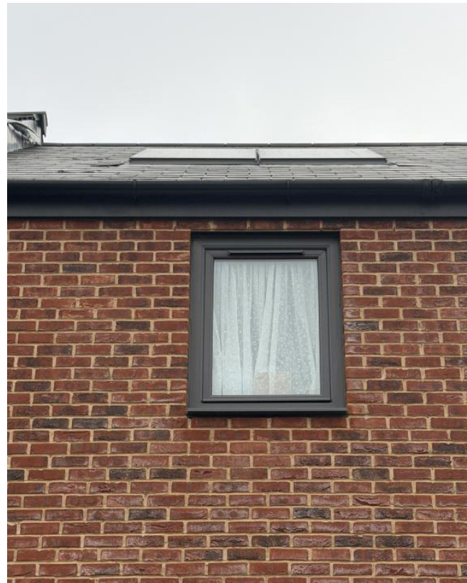
Close view of the roof.
