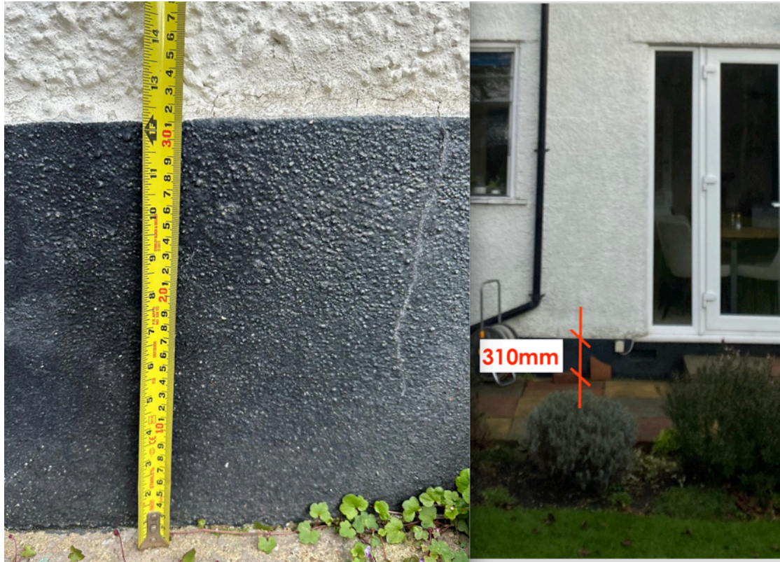
Figure 4.1 Existing House Floor Level Above Site Level
