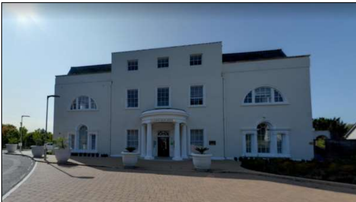
Figure 3: Site – View of front forecourt
