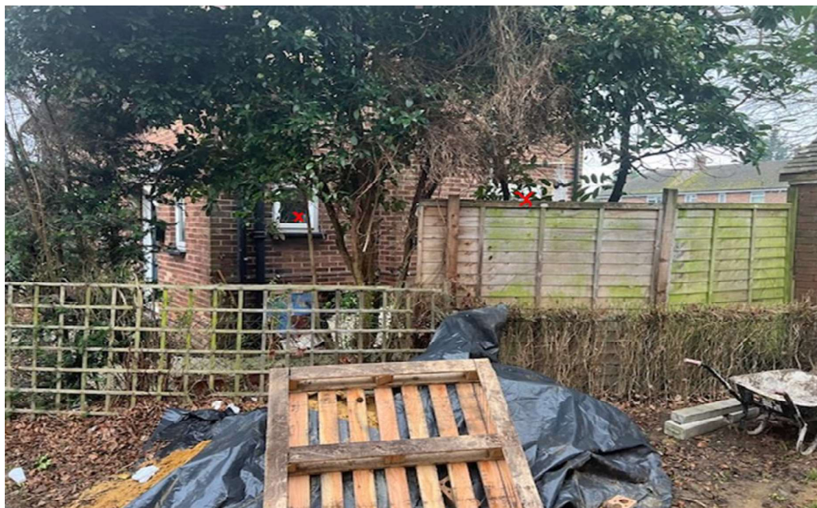
Figure 5: 11 Oak Avenue ground Floor side windows
