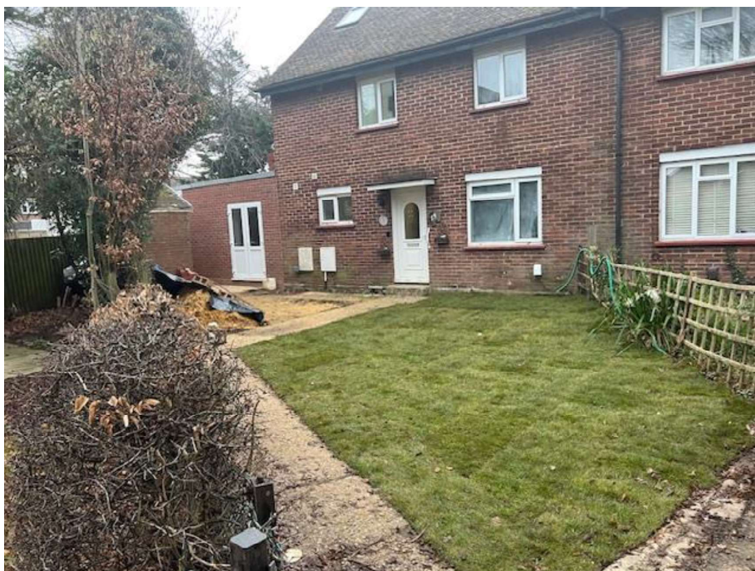
Figure 3: Front Elevation of the Property
