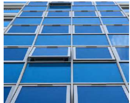
Aluminium clad curtain walling
