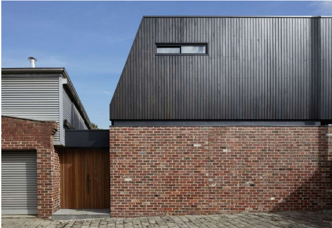
Red Brick Plinth / Dark Metalwork cladding
