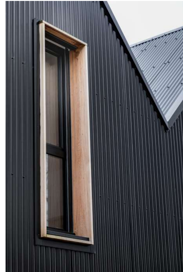
Ribbed metalwork cladding profile
