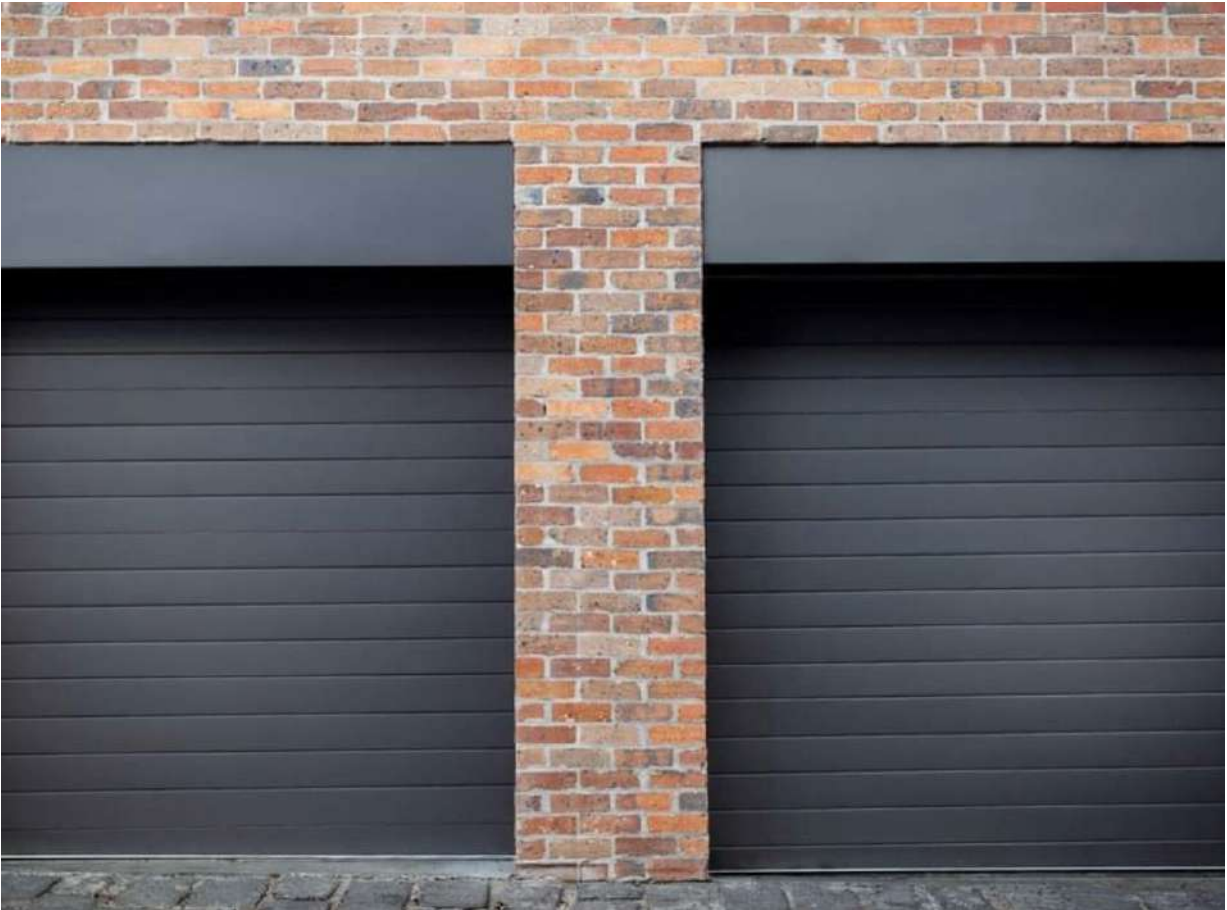
Accentuated Lintels / brick piers - Garage Block
