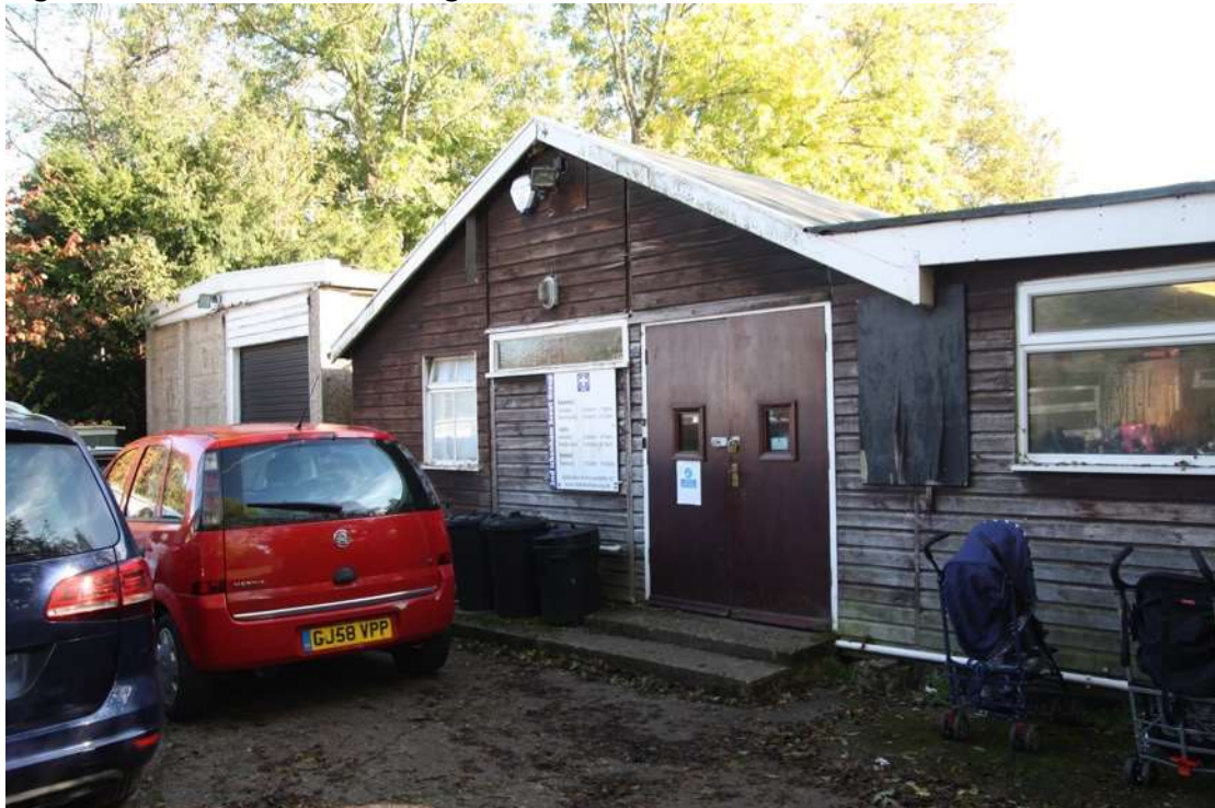
Fig 6: Existing scout-hall located east of the site to be demolished.
