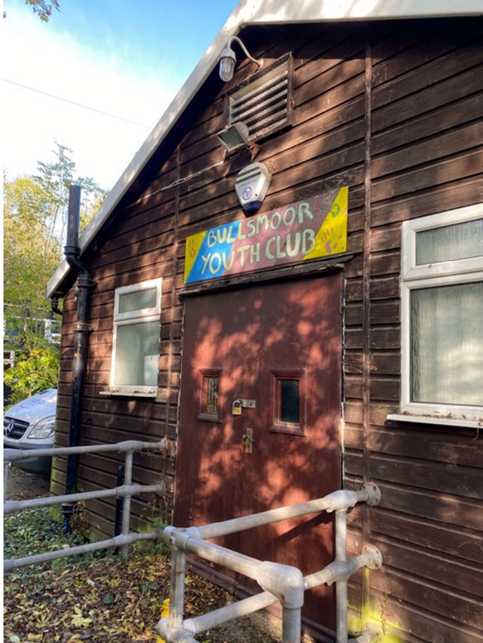
Fig 3: Front elevation and access to the existing scout-hut. Proposed to be demolished.
