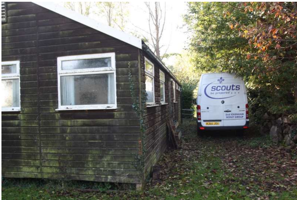
Fig 4: Side view of the existing scout-hut.
