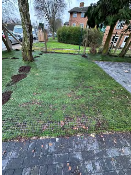
Photograph 13: B & X Construction Ltd Supplied Photograph – Tensar SS20 covering soft landscaped area to front of building, photograph taken on 01.02.2025.
