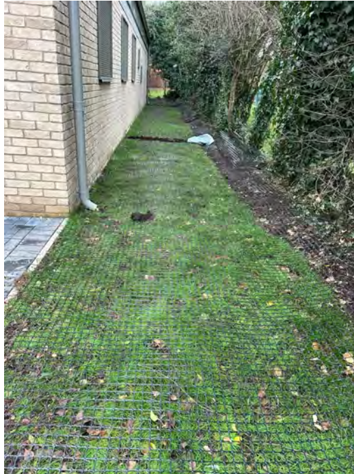
Photograph 11: B & X Construction Ltd Supplied Photograph – Tensar SS20 placement to side of building, photograph taken on 01.02.2025.
