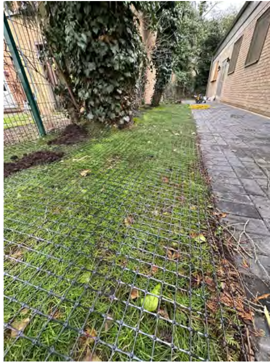
Photograph 15: B & X Construction Ltd Supplied Photograph – Tensar SS20 placement to Soft Landscaped Area to side of the building and Block Paving, photograph taken on 01.02.2024.
