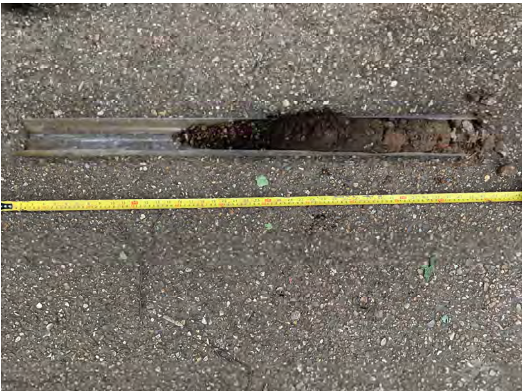
Photograph 4: Encountered ground conditions. WS01 0.0 – 1.0mbgl.
