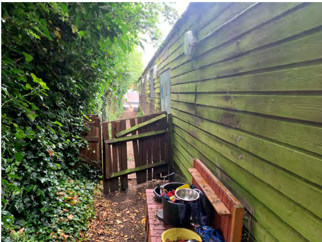
Photograph 2: Northern section of site, looking east.
