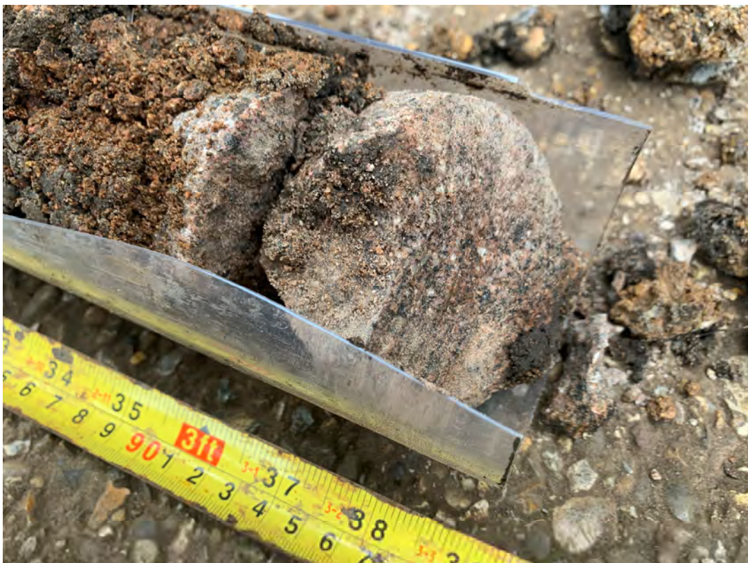
Photograph 8: Concrete encountered within base of WS05, 0.9 – 1.0mbgl.
