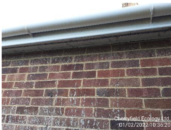
Figure 17: Example of brick work in good condition and tight-fitting soffits on B1b
