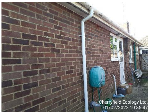
Figure 16: Further example of soffits flush against walls of B1a
