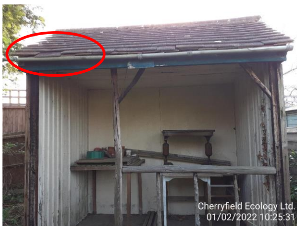
Figure 20: Small number of gaps in roof tiles in B3
