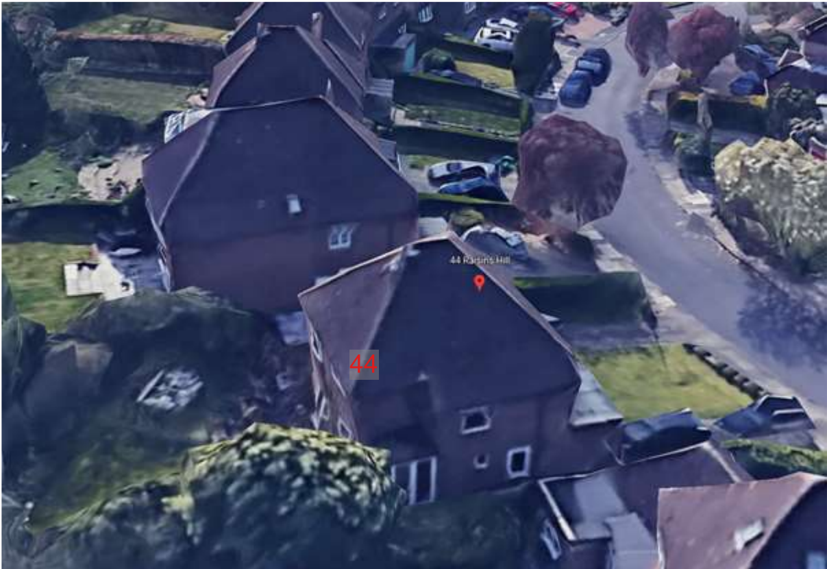
VIEWS SHOWING NEIGHBOURING PROPERTY 42 RAISINS HILL EXTENDING OUT FURTHER THAN APPICATON PROPERTY 44 RAISINS HILL
