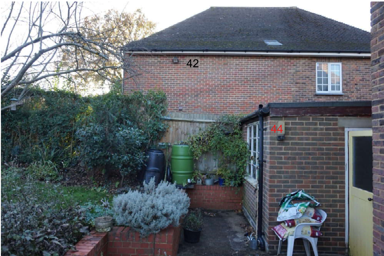
VIEWS SHOWING NEIGHBOURING PROPERTY 42 RAISINS HILL EXTENDING OUT FURTHER THAN APPICATON PROPERTY 44 RAISINS HILL
