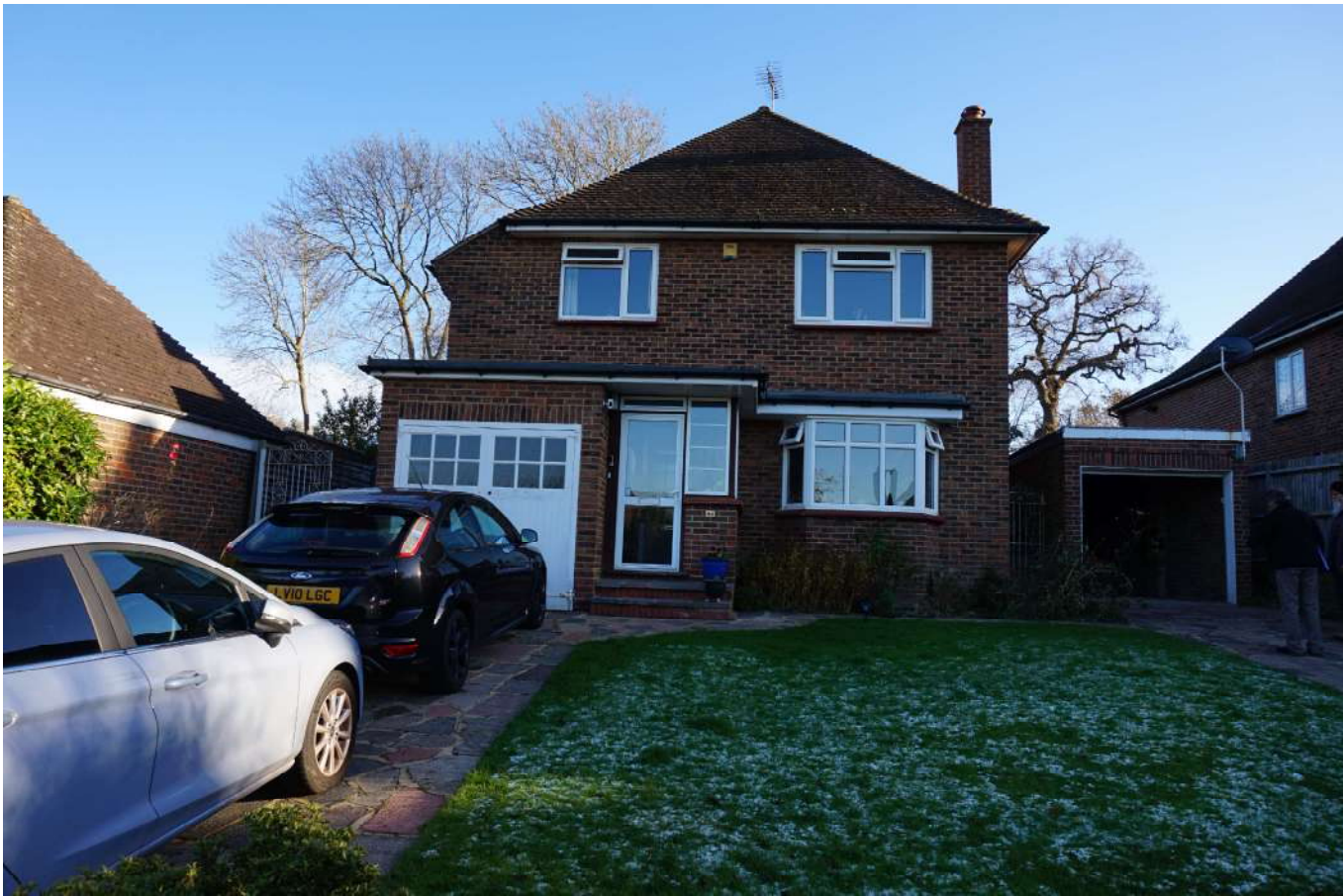
VIEW - FRONT (STREET)
