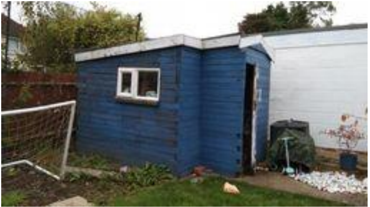
5 View of shed and outbuilding at adjoining property
