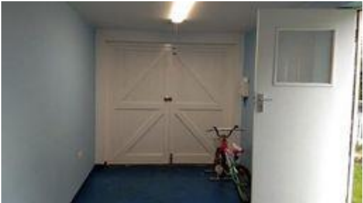
6 Garage door from inside the garage
