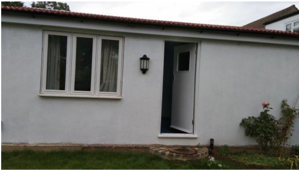
7 South East Side View of the Garage
