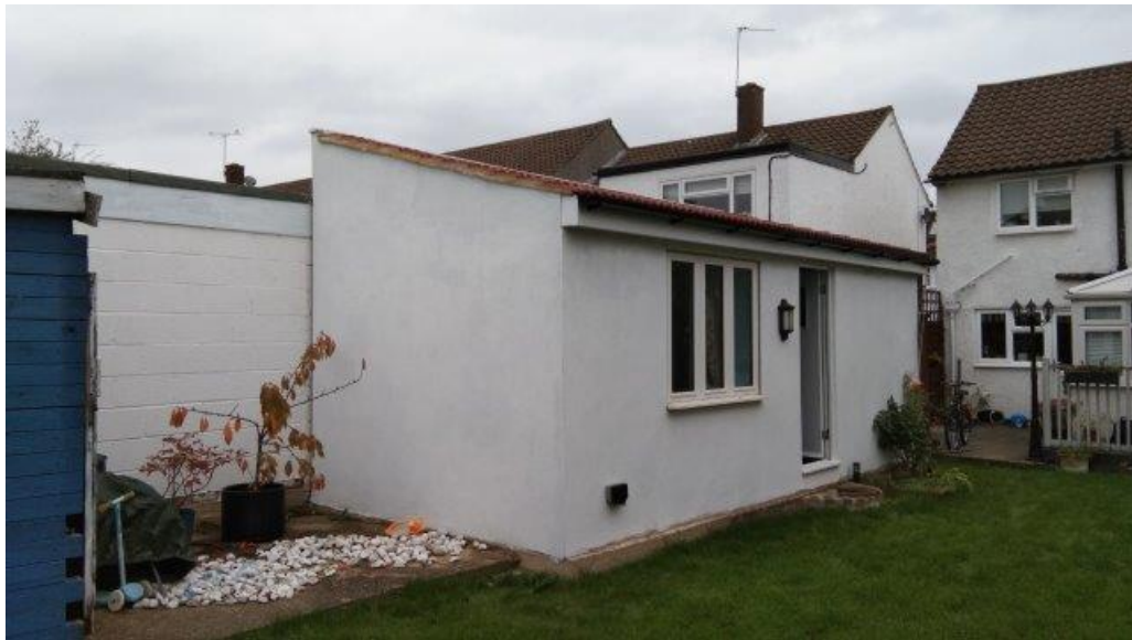
8 South East side view of the Garage
