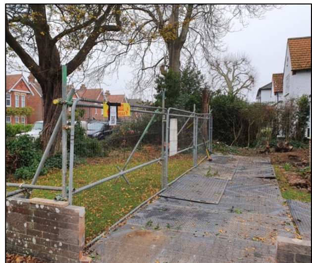
GP2: Tree protection barriers & trackmat ground protection
