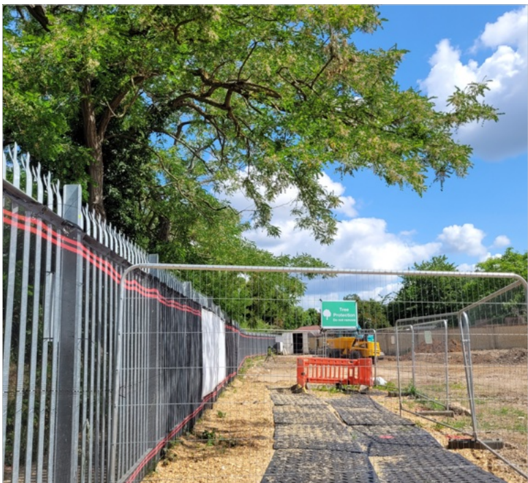
Ground protection in place
