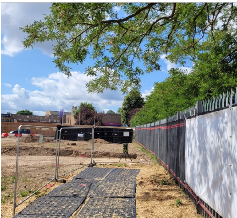
Ground protection in place
