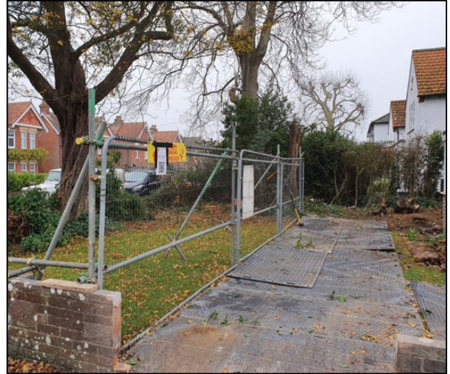
GP2: Tree protection barriers & trackmat ground protection
