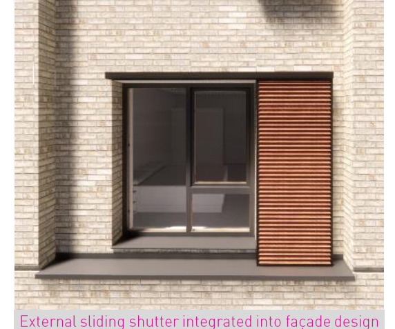
External sliding shutter integrated into façade design
