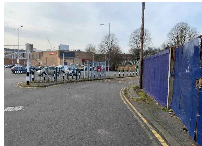
3 – ACCESS ROAD WITH HOARDED SITE AND PUBLIC CAR PARK
