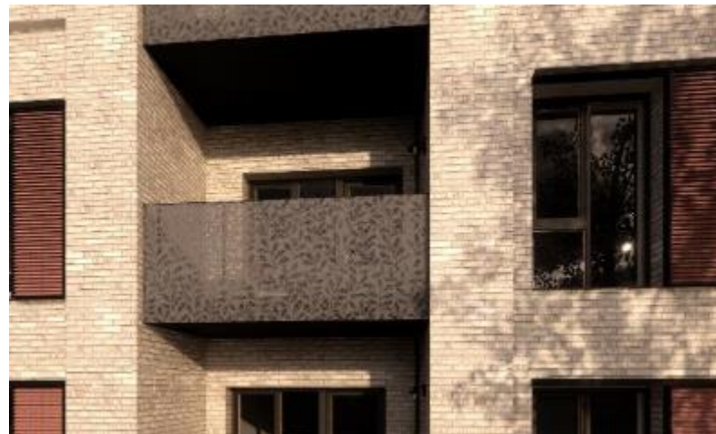
Detail of the rear elevation with perforated metal sheet balustrade with leaf pattern
