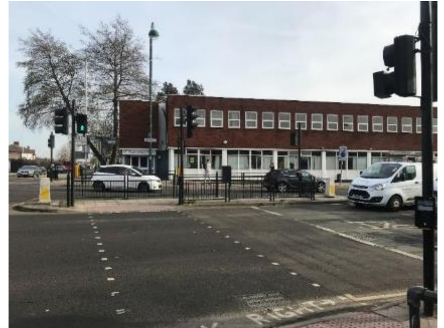
1 - VIEW WEST LOOKING FROM THE HIGH STREET
