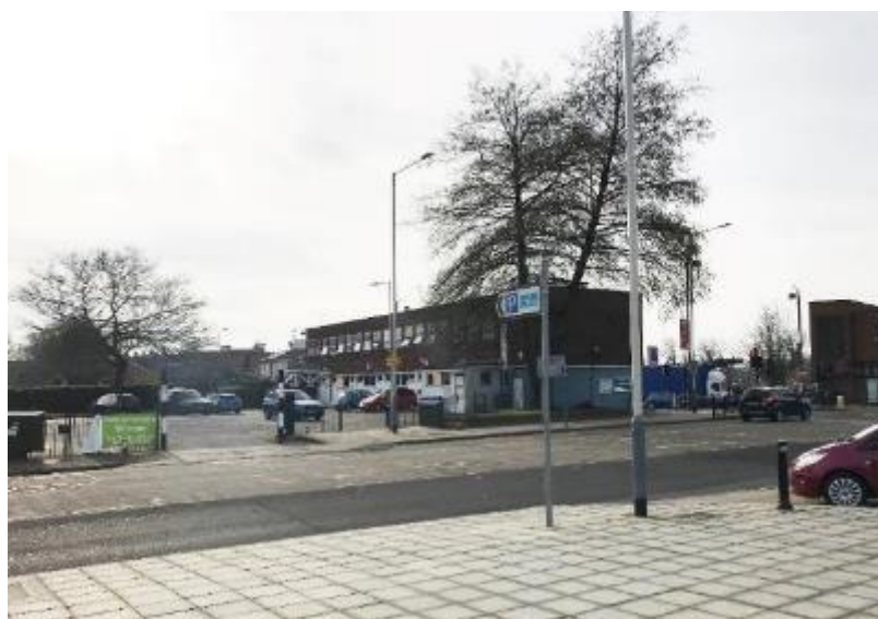
17 – VIEW OF THE EXISTING LIBRARY FROM THE NORTH SIDE OF FALLING LANE
