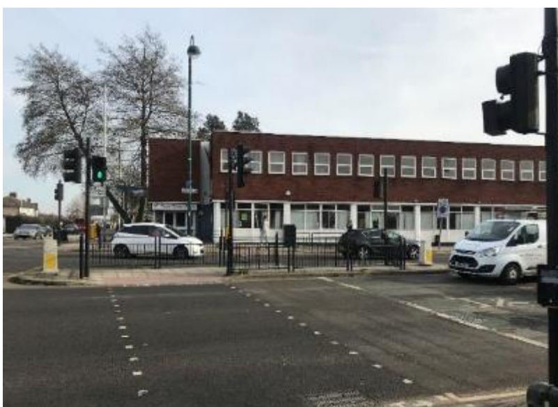
5 – VIEW TO EXISTING LIBRARY FROM HIGH STREET JUNCTION
