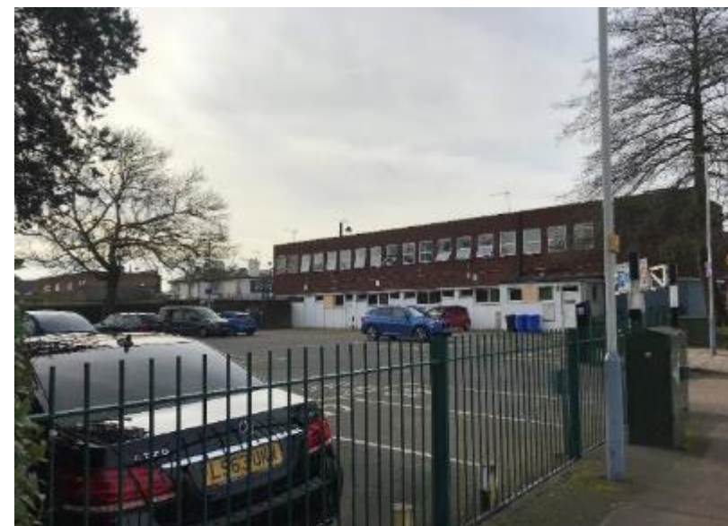
3 – VIEW TO EXISTING LIBRARY & CAR PARK FROM FALLING LANE
