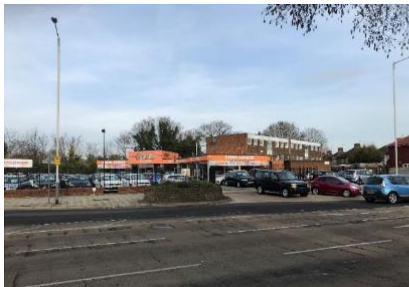
13 – VIEW OF FLC CARE SALES FROM FALLING LANE
