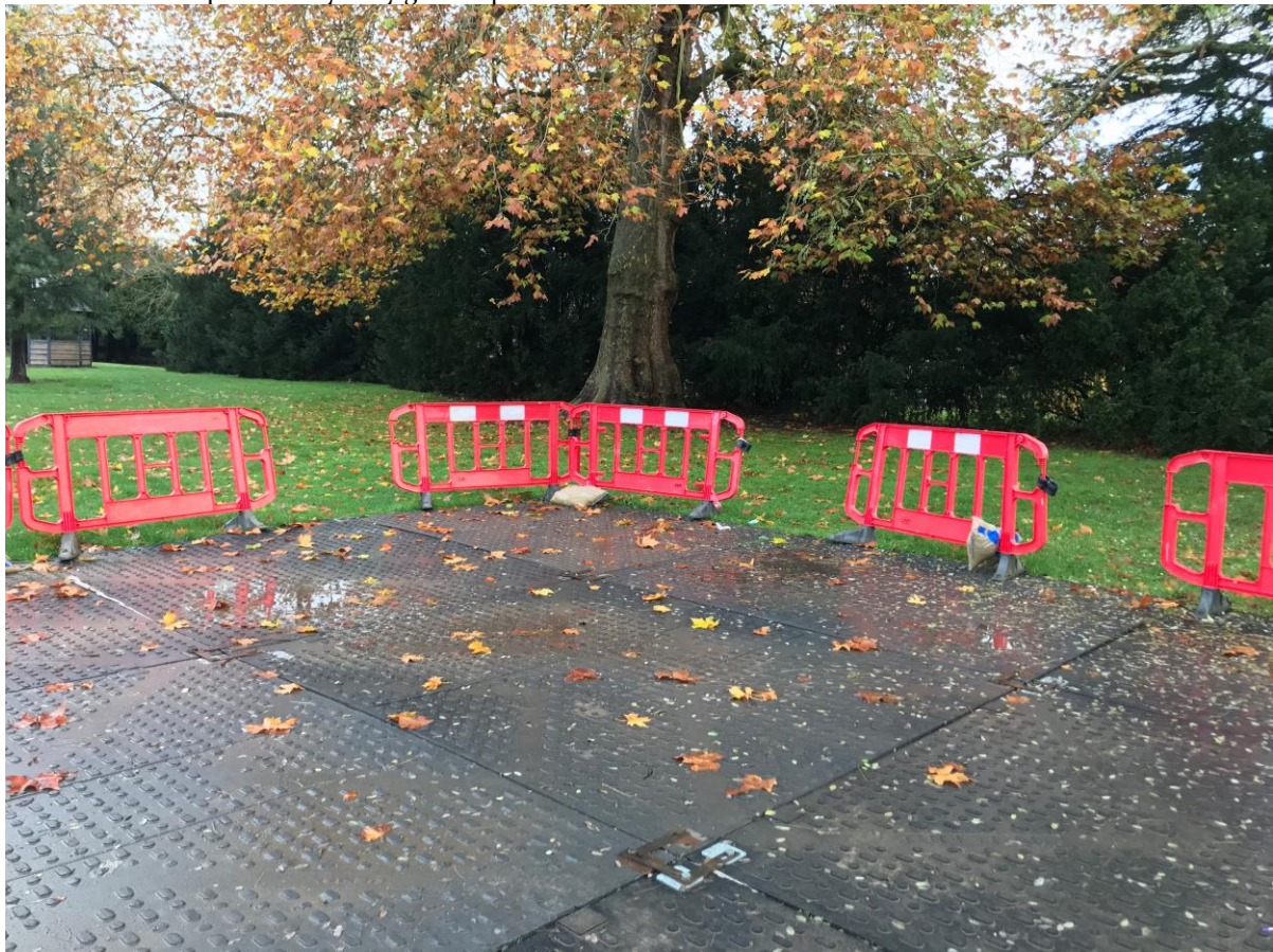
Photo 2. An example of heavy-duty ground protection.
