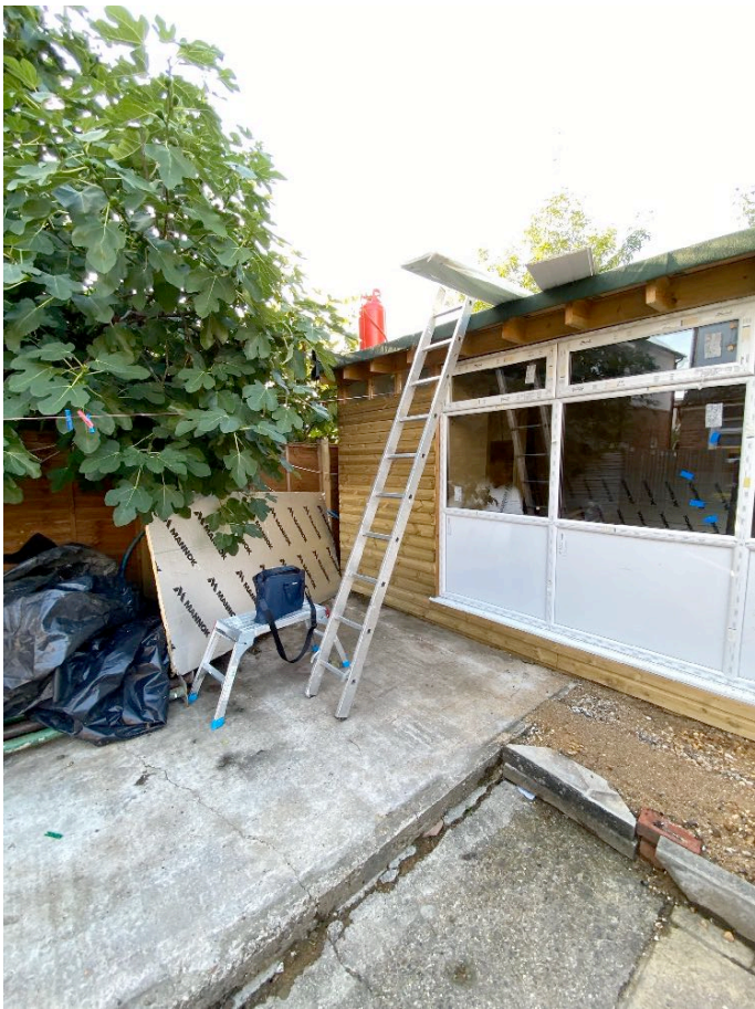
1. View looking West towards the as-built and western boundary with no. 3 Cherry Orchard. Note there is landscaping and screening between the two properties.
