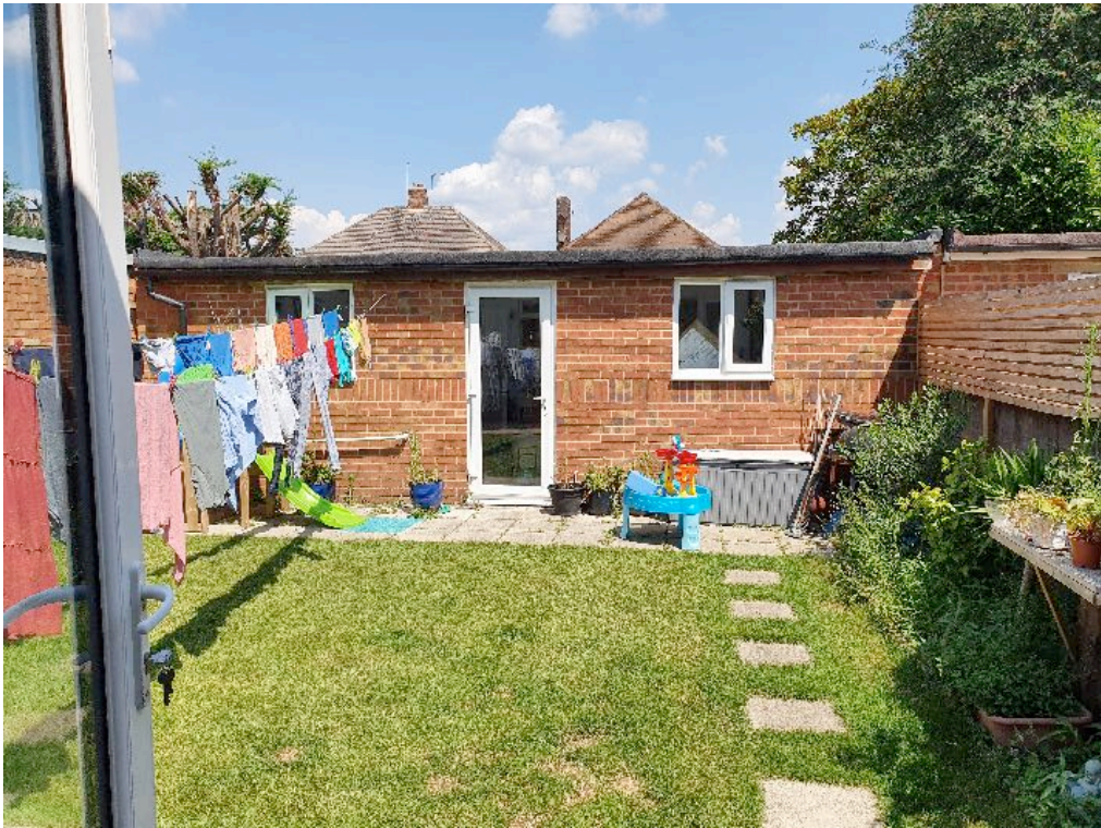
12. View looking North-East, towards the rear of property No. 39 Belmore Avenue garden and outerbuilding.
