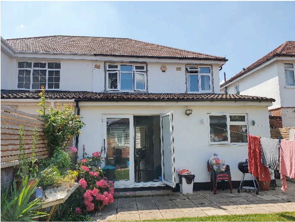
9. View looking South-East towards the rear of the property No. 39 Belmore Avenue showing the Patio.
