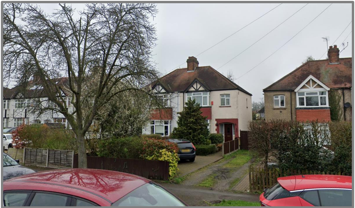
Figure 1: Existing dwelling, access and parking via Long Lane
