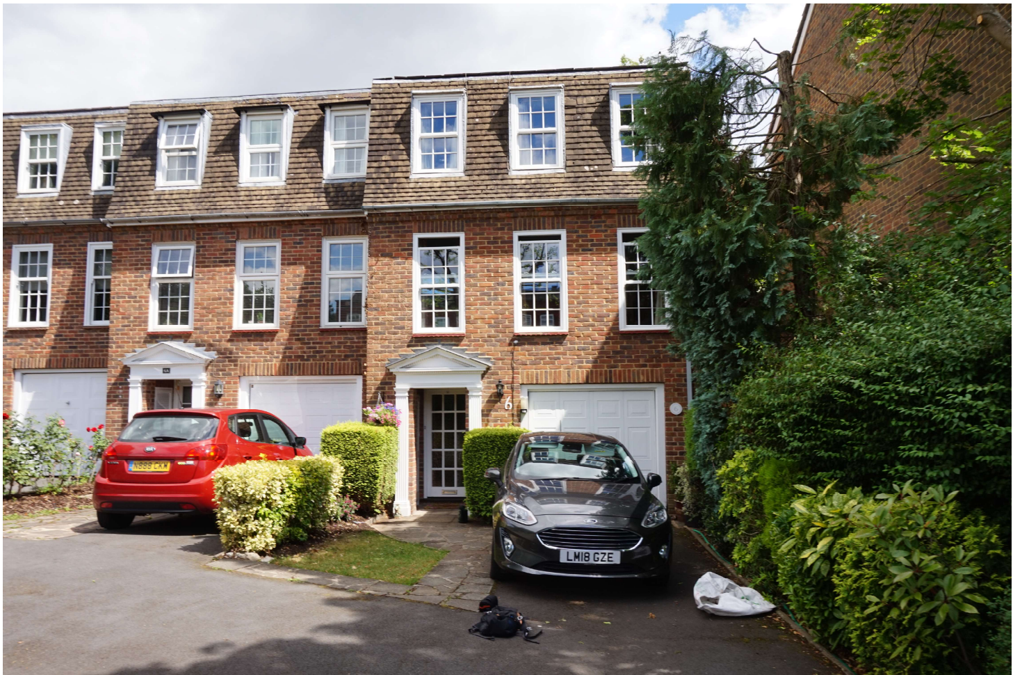
VIEW - FRONT (STREET)
