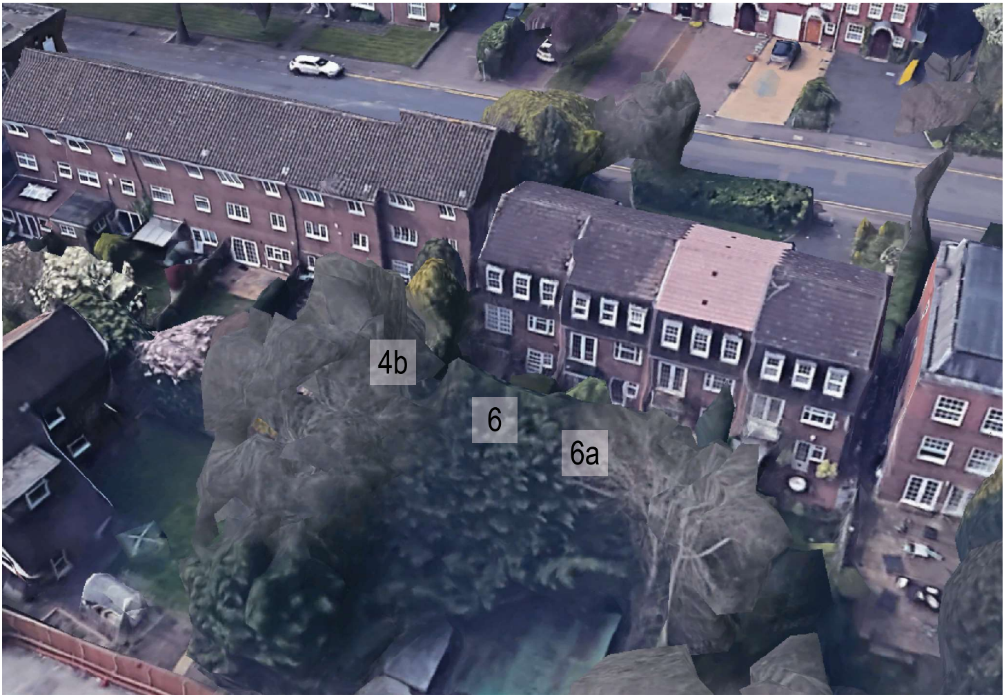
AERIAL VIEW - REAR
