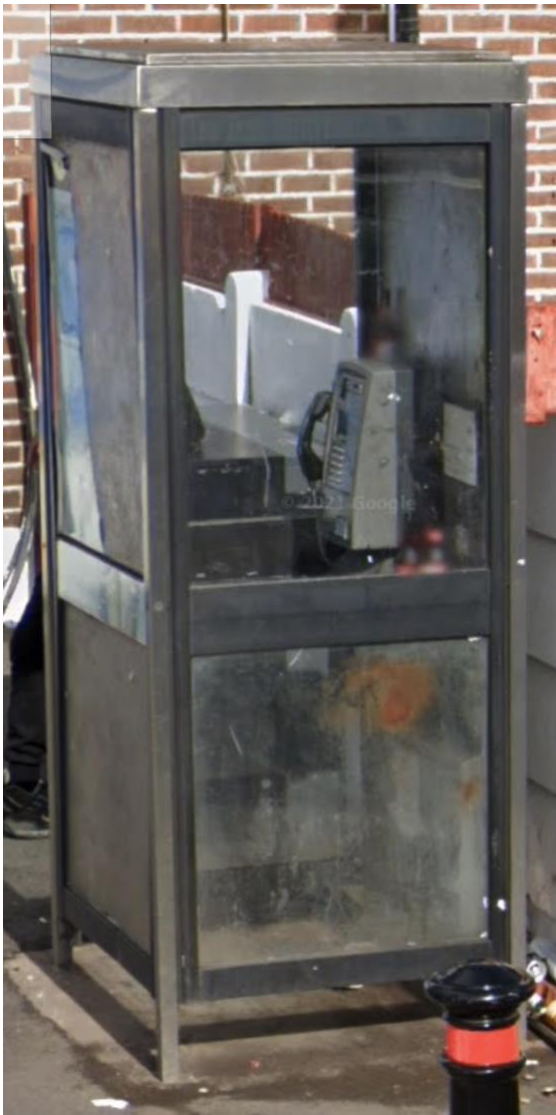
REMOVAL 1 – PHOTOGRAPH OF KIOSK
