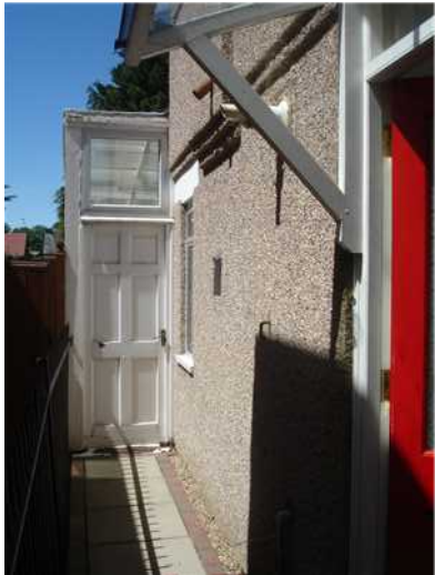
Views from side alleyway
