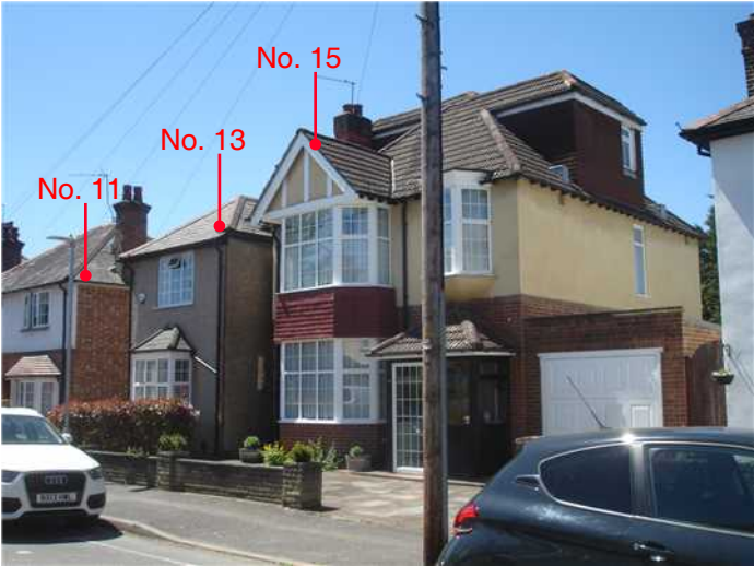
Views from Hilliard Road
