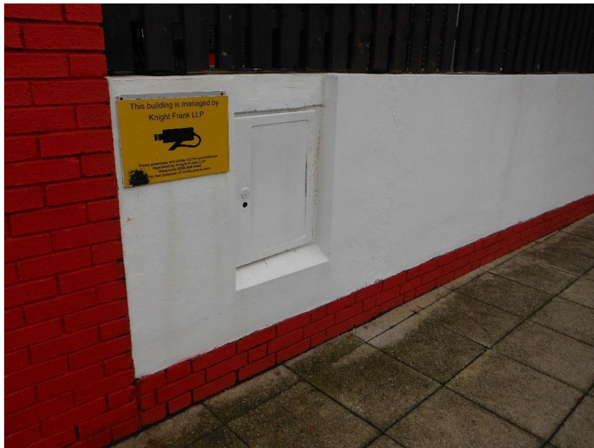
Photo 2. UST Offset Fill Point
