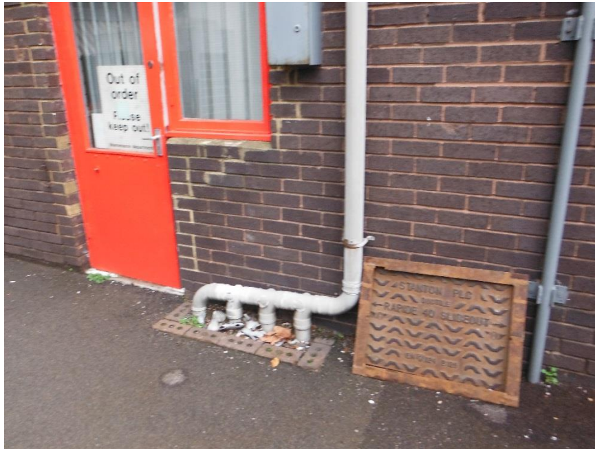
Photo 3. Former Vent Pipes Associated with Former Fuel Filling Operations
