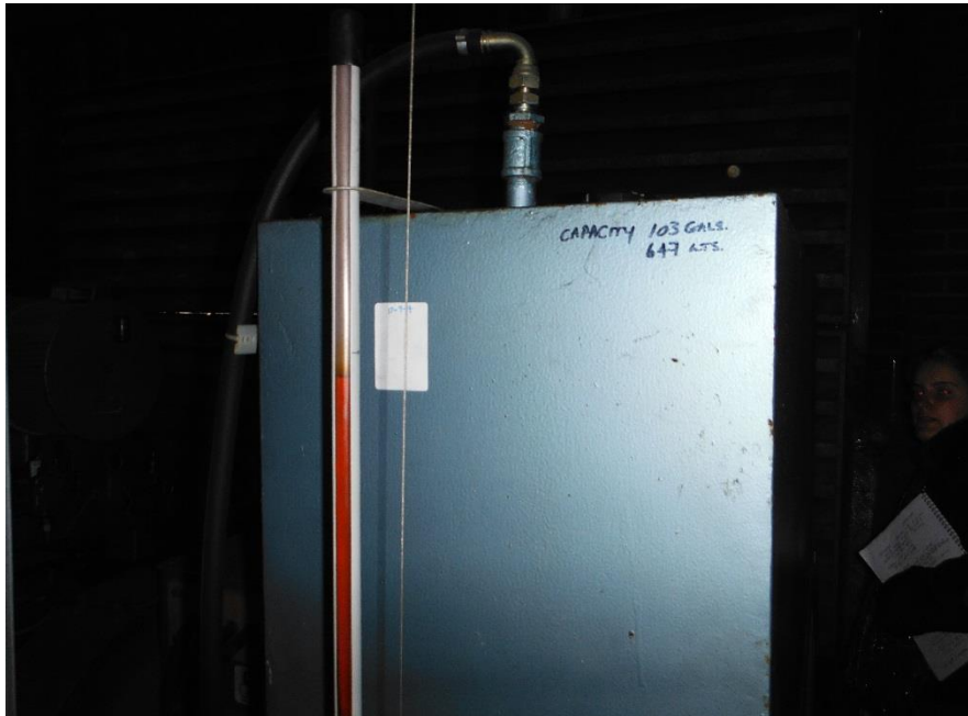
Photo 5. 650 Litre Day Tank for Building 3 Generator (fed from UST)
