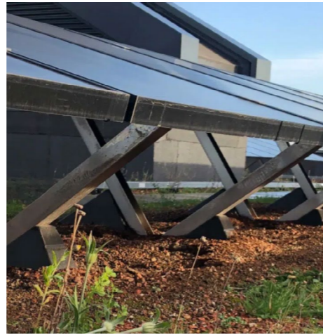
PV panels on brown roofs
