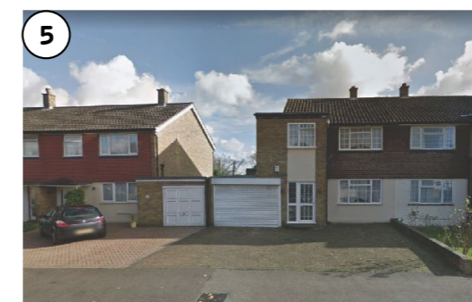
Hitherbroom Road 1960's Houses
