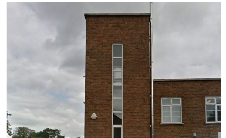
Vertically expressed staircase fenestration
