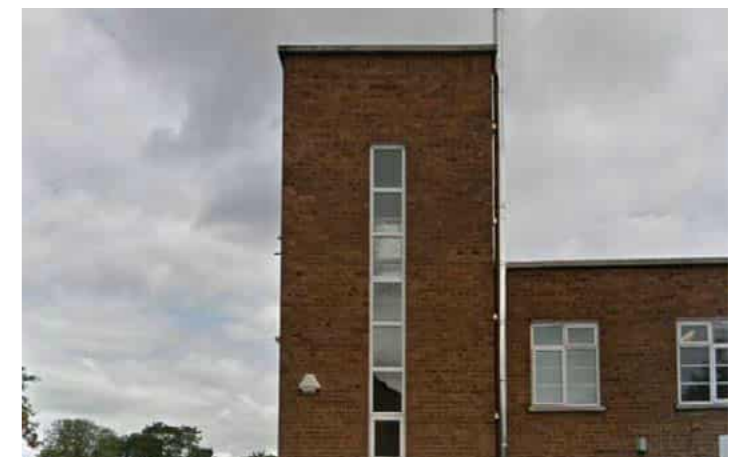
Vertically expressed staircase fenestration
