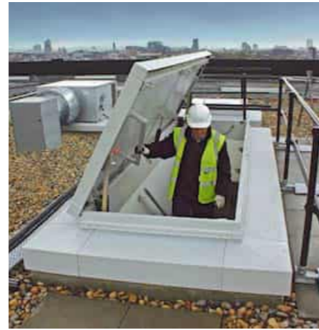
'Coffin' roof hatch access with stair up to hatch
