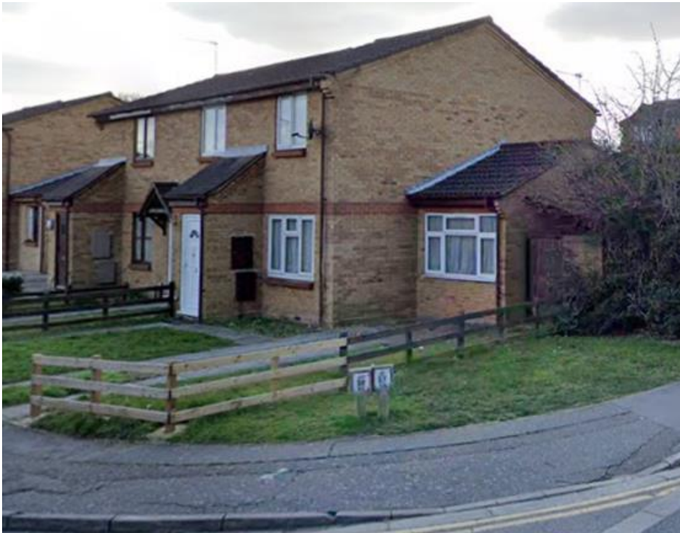
Image 9 - View of 66 Gade Close from the site, front elevation
