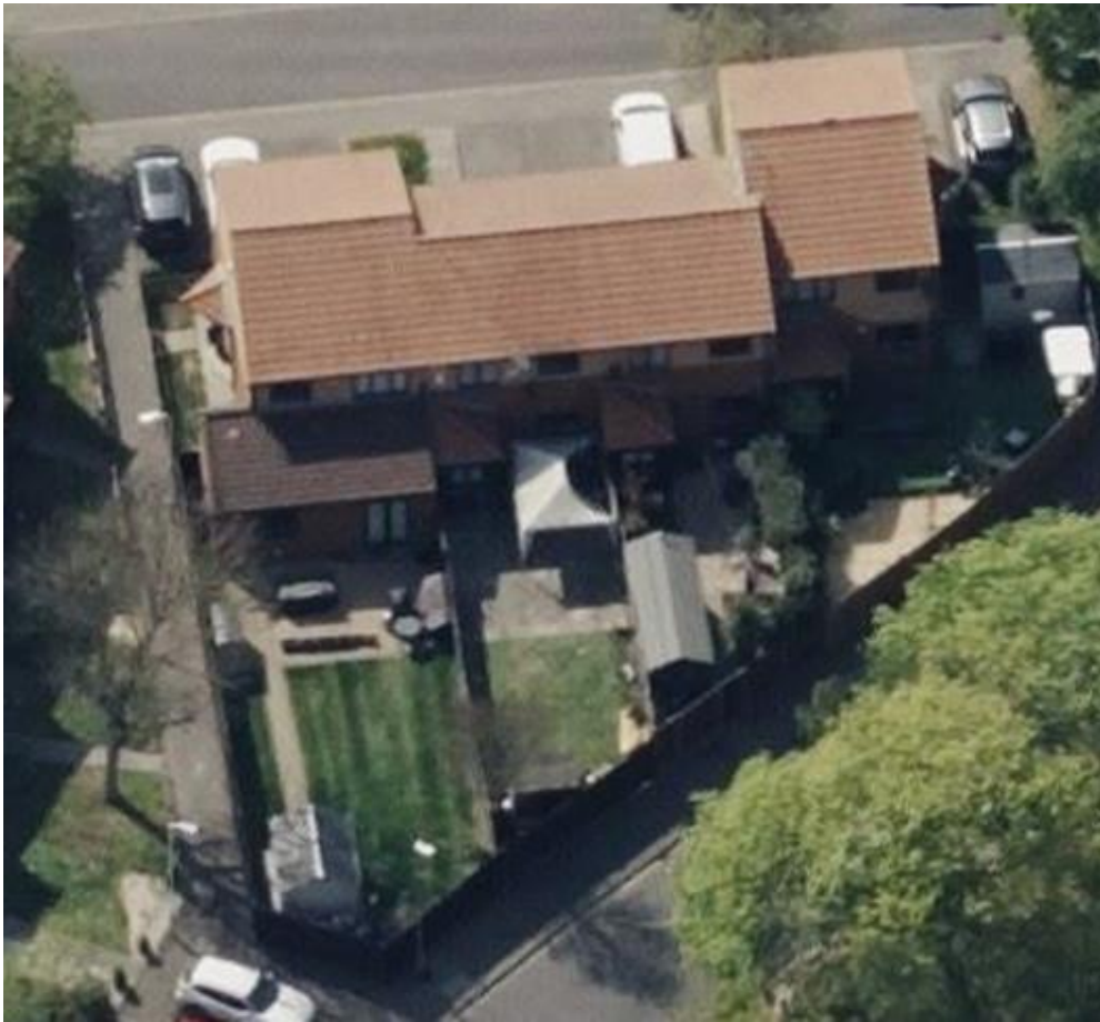
Image 12 - Aerial view of 127-133 Avondale Drive, rear elevations
