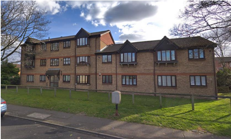
Image 8 - Street view of 1-17 Clivesdale Drive, front elevation
