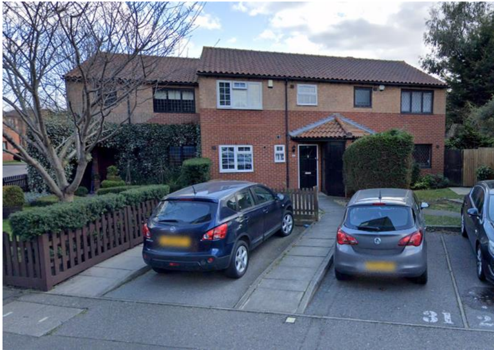
Image 11 - Streetview of 29 – 33 Avondale Drive
