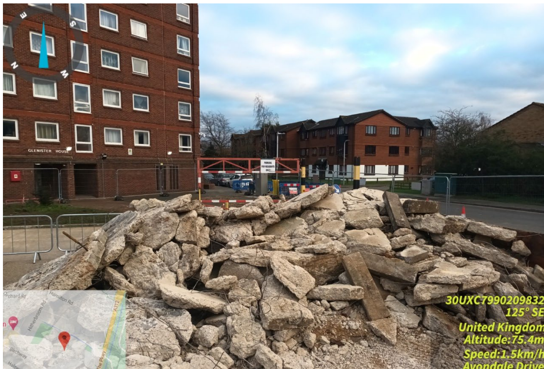
Segregated Concrete Stockpile
