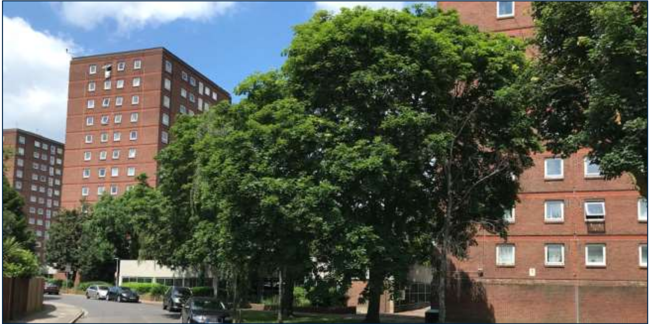
Figure 10: Looking west along Avondale Drive
