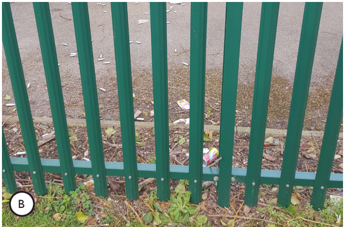
Fence and planting preventing access from the estate to Hitherbroom Park
