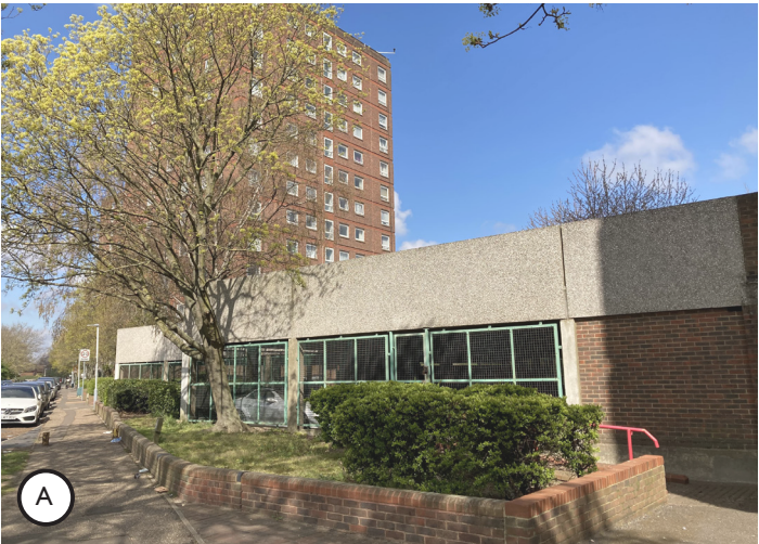
Mesh enclosure to parking structures onto Avondale Drive
