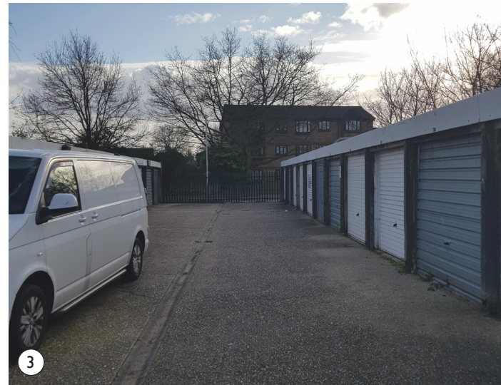
Garages in west of site
