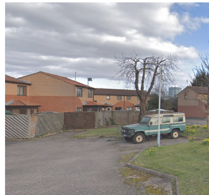
Housing developments on Avondale Drive
