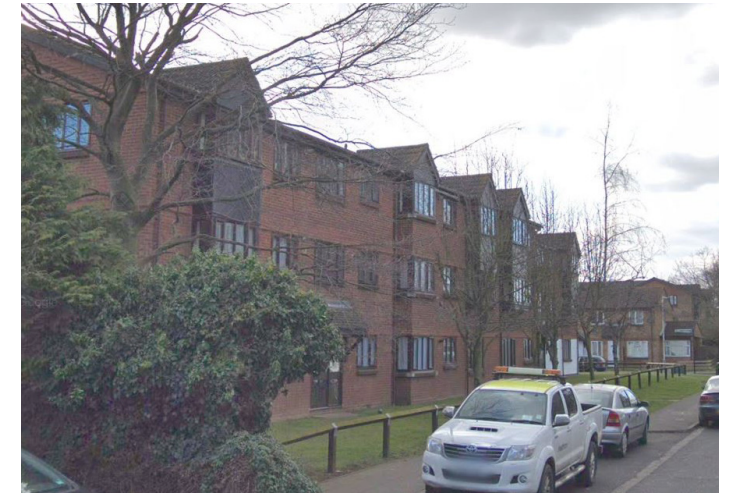
Housing developments on Avondale Drive
