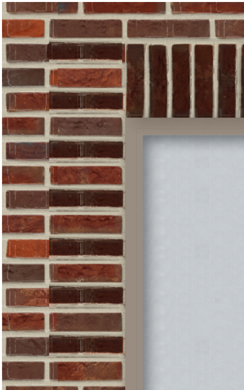
Alternating brickwork detail
