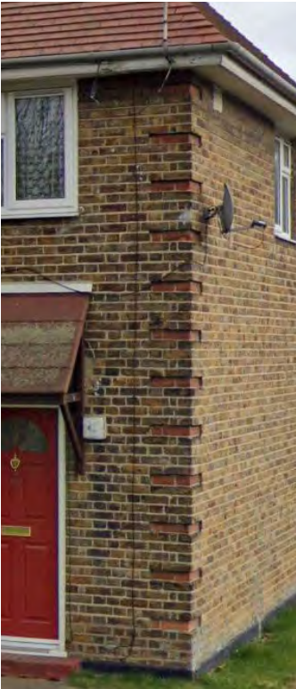
Existing brick quoin details
