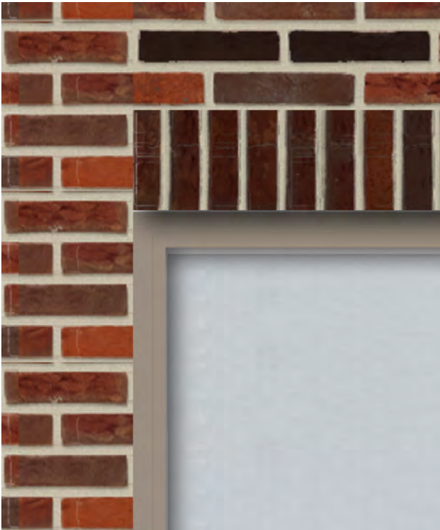
Materiality coming together on front facade; red brick with white mortar, alternating red and claret bricks, claret soldier course bricks
