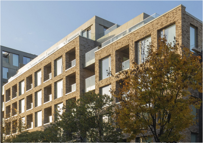
Building designed to break up massing (Pentonville Road, PTE)
