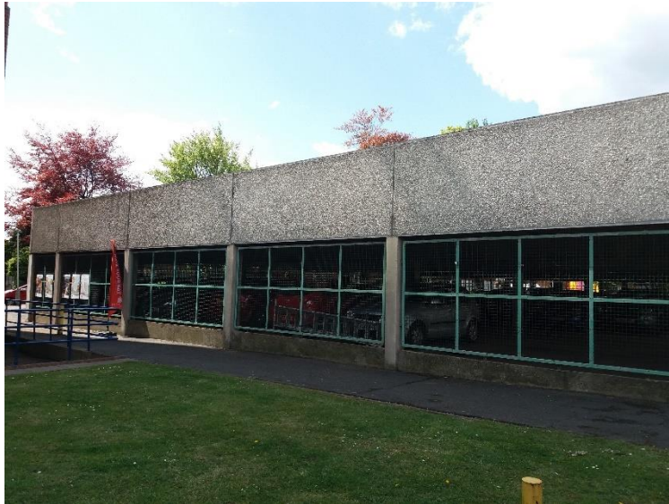
Figure 4.6 View of building 4 from the north
