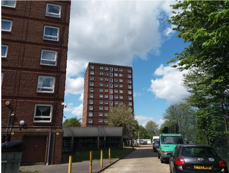
Figure 4.5 View of building 5 and 3 from the east of site
