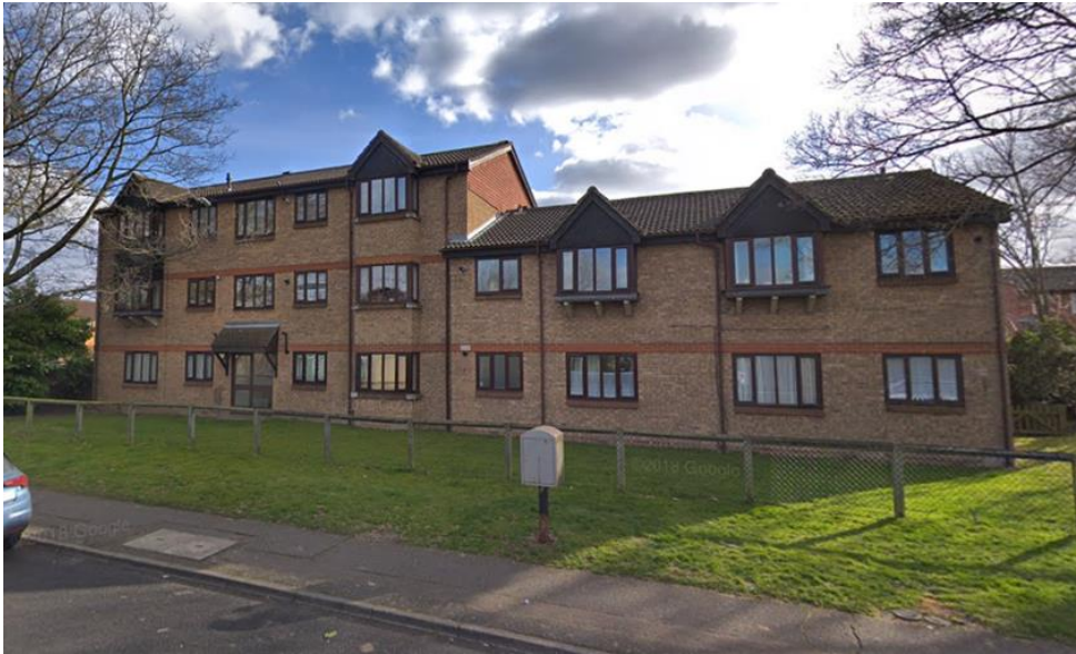
Image 9 - Street view of 1-17 Clivesdale Drive, front elevation
