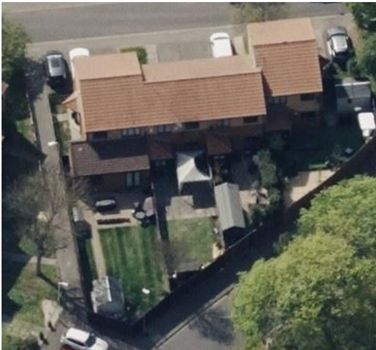
Image 13 - Aerial view of 127-133 Avondale Drive, rear elevations
