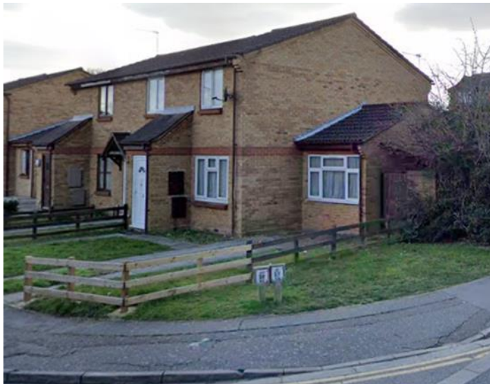
Image 10 - View of 66 Gade Close from the site, front elevation
