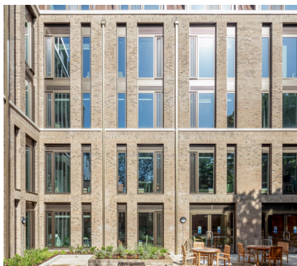
Vertical articulation of windows contributes to the facade design
