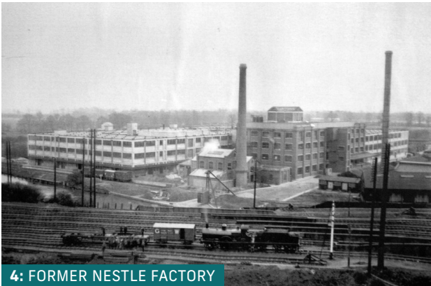
4: FORMER NESTLE FACTORY
