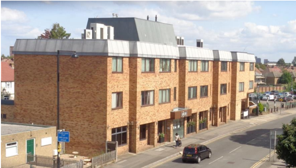
Image 6 - Site photo of 18-22 Pump Lane, Front elevation
